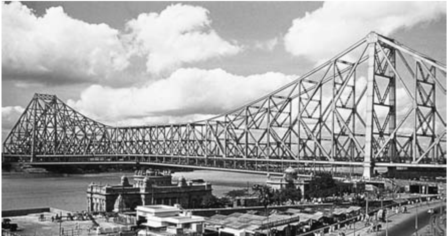
Figure 1.11 Howrah Bridge, Kolkata, India.
