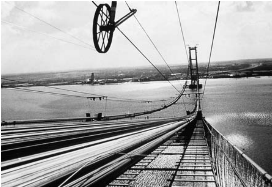
Figure 1.23 Cable Spinning for Humber Bridge.
