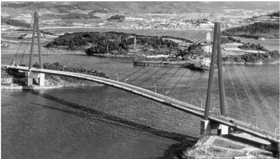
Figure 1.29 Jindo Bridge, South Korea.
