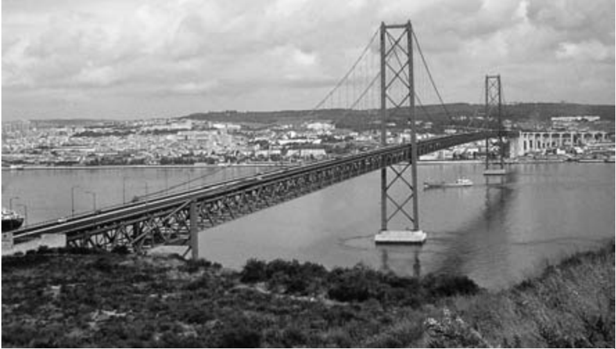
Figure 1.20 Salazar Bridge over the Tagus, Portugal (1964).
