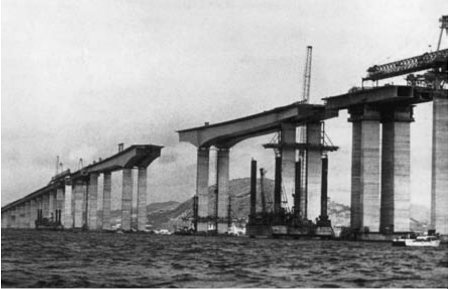
Figure 1.39 Rio Niteroi Bridge, Brazil.
