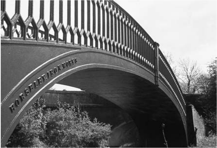
Figure 1.5 Arch Bridge over Oxford Canal, England (1832–34).
