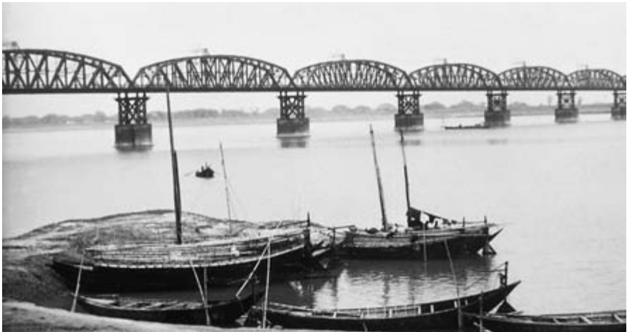
Figure 1.12 Hardinge Bridge, India.
