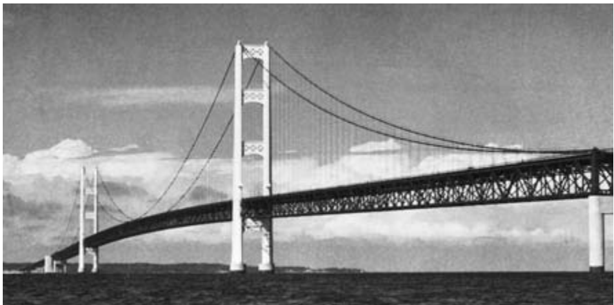
Figure 1.18 Mackinac Bridge, Michigan (1957).
