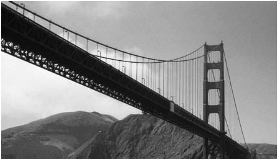
Figure 1.16 Golden Gate Bridge, San Francisco (1937).
