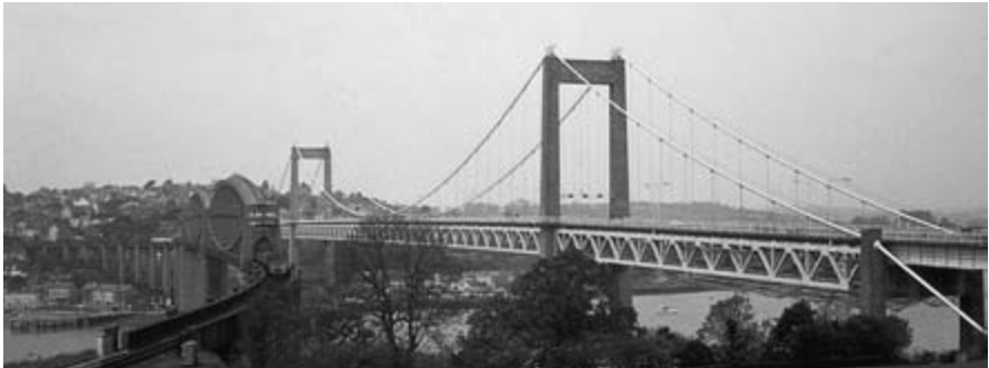
Figure 1.17 Tamar Suspension Bridge, England (Brunel's bridge can also be seen).
