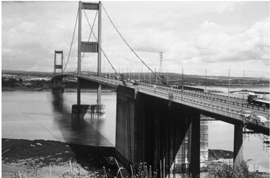
Figure 1.21 Severn Road Bridge, England (1966).
