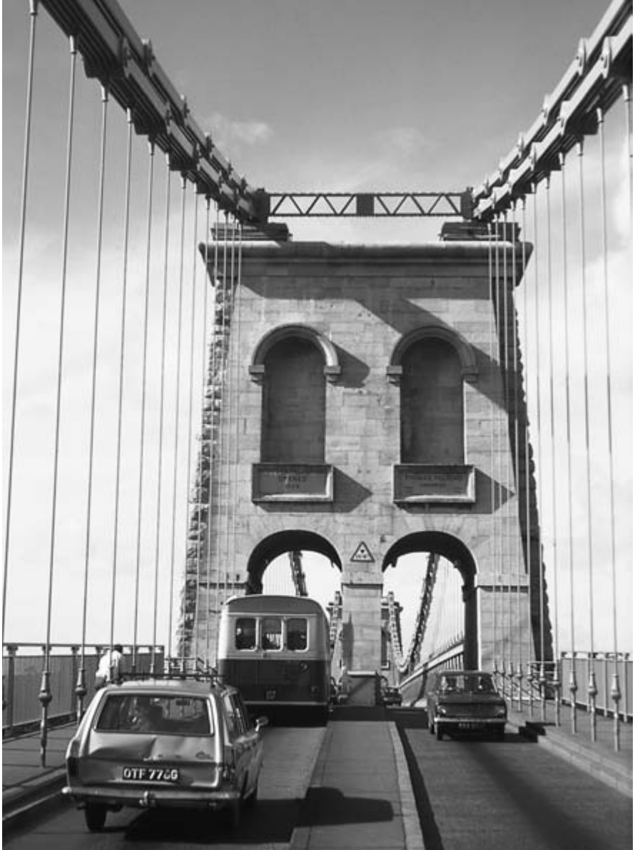
Figure 1.4 Suspension bridge across the Menai Straits, Wales (1819–26).
