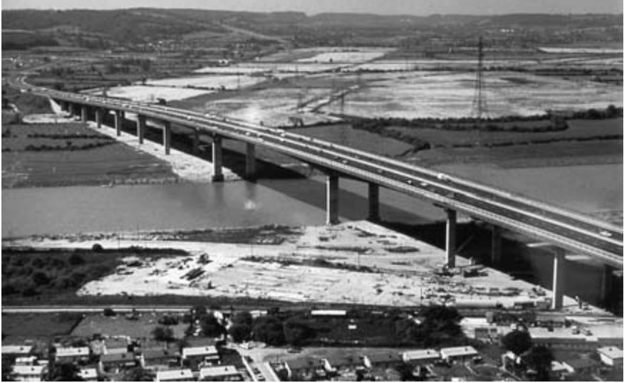
Figure 1.34 Avonmouth Bridge, England.
