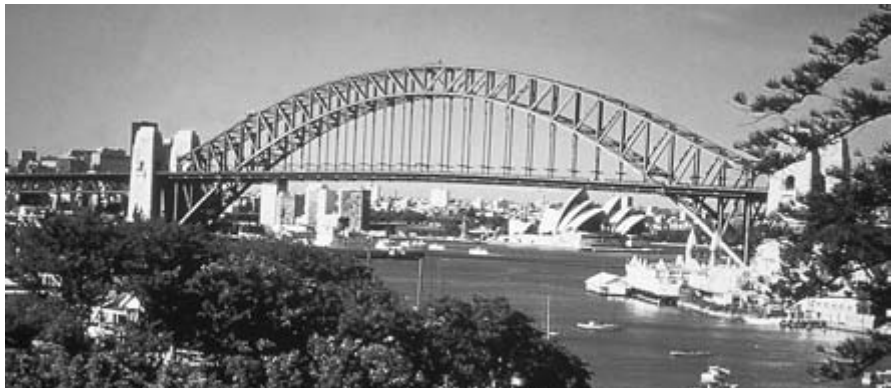
Figure 1.14 Sydney Harbour Bridge, Australia (1923–32).
