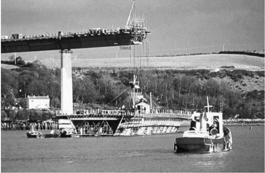
Figure 1.33 Milford Haven Bridge during construction.
