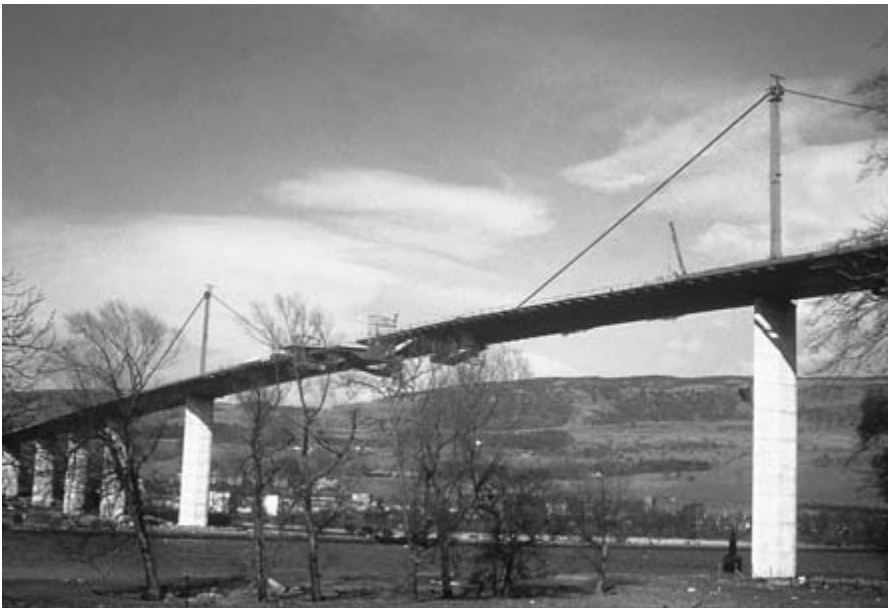
Figure 1.27 Erskine Bridge, Scotland (1971).
