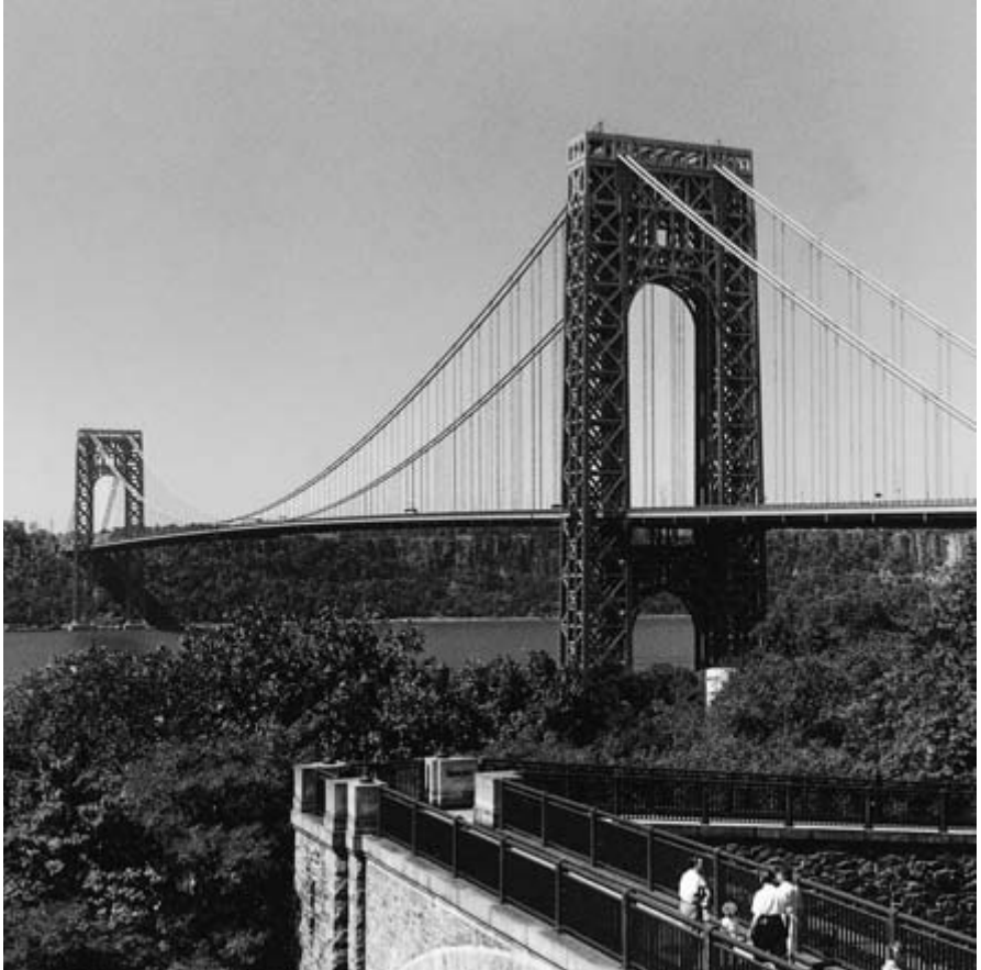
Figure 1.15 George Washington Bridge, New York (1931).
