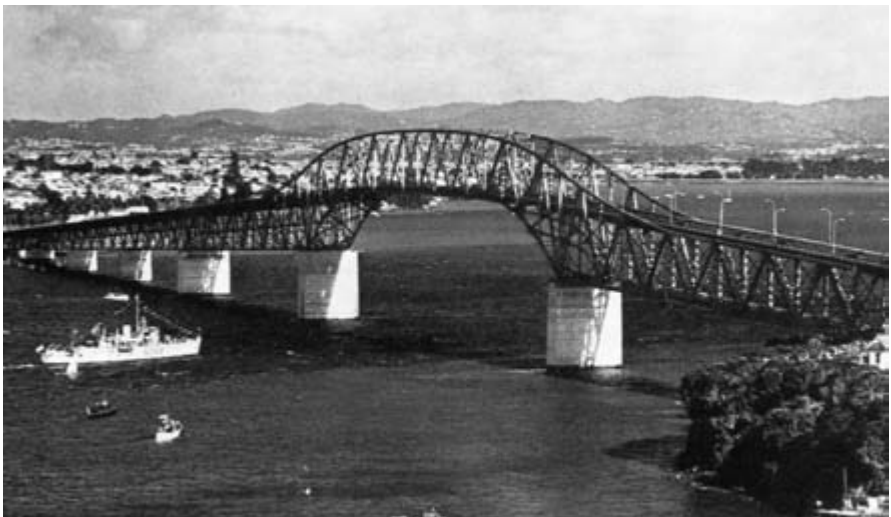
Figure 1.32 Auckland Harbour Bridge, New Zealand (1969).
