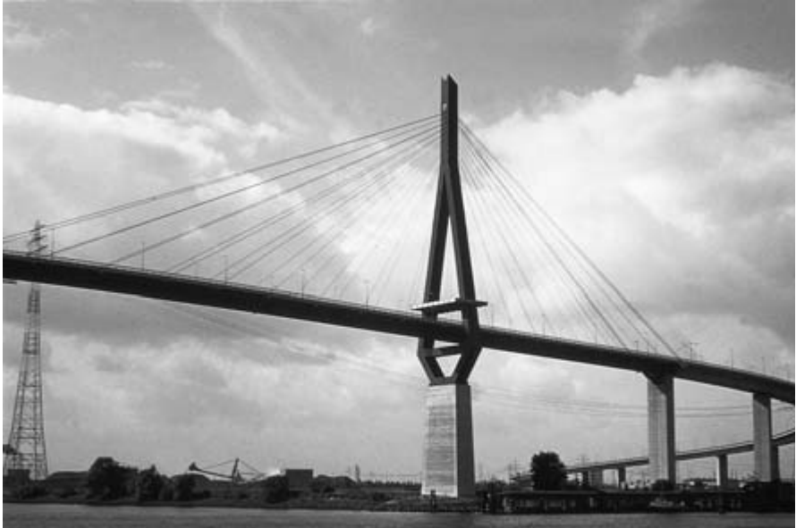
Figure 1.28 Kohlbrand Bridge, Hamburg, Germany (1974).
