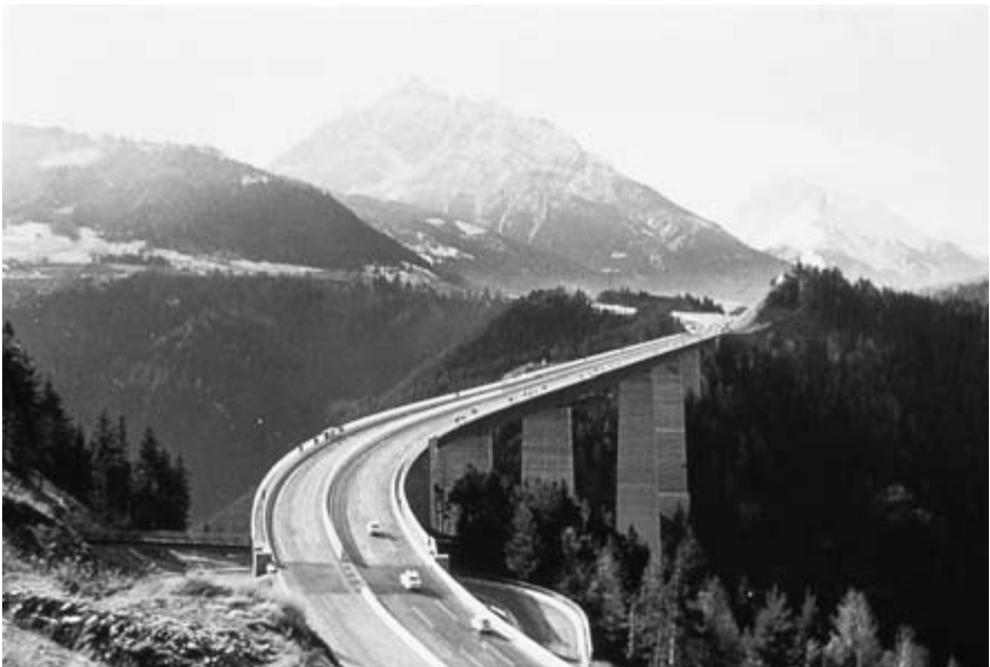
Figure 1.35 Europa Bridge, Italy.
